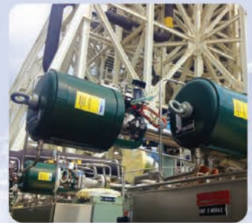
Trimteck designed valves for LOX and IPA service on the Chemical Steam Generator at NASA's A-3 Test Facility
