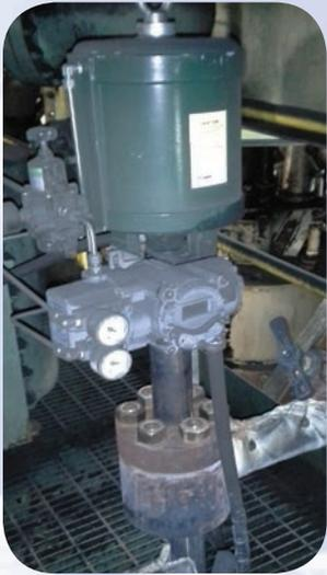
*Installation was straightforward. We spun the actuator 180-degrees to make the positioner more accessible and welded the valve in place.*
